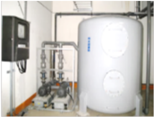
Construction of rainwater recovery system
