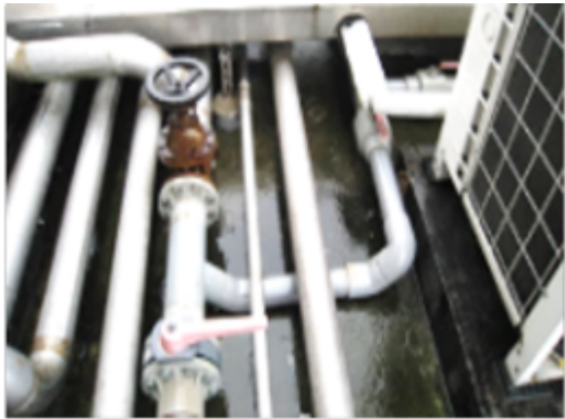
Integration of rainwater recovery systems across all factories
