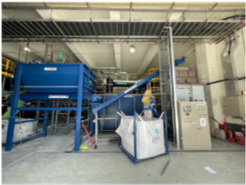
Installation of additional sludge drying equipment
