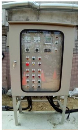
Discharge monitoring and control panel
