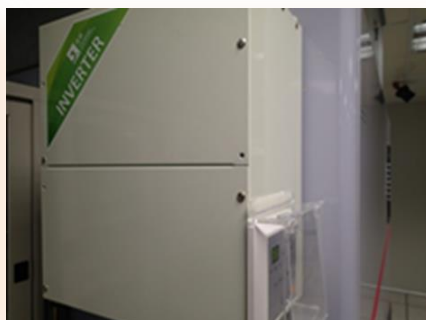
Air conditioner in MDF computer room changed to inverter
