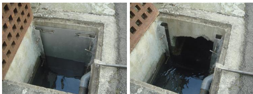
↑Rainwater gutter installed with water gate for recycle and treatment in stimes of abnormal water quality↑
