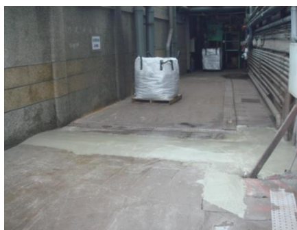
↑Sludge Storage Zone installed with water division pier
